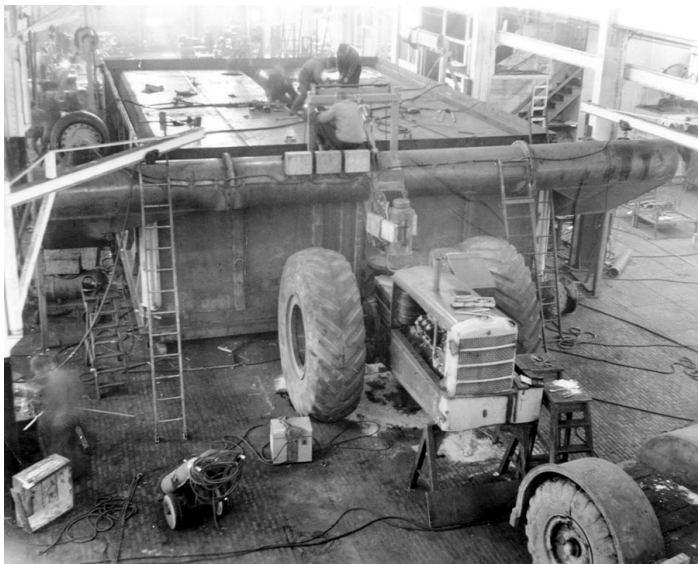
Figure 4. Tournalayer No. 2, Peoria, Illinois, Concrete house casting and laying system in the process of construction, 1946, Courtesy LeTourneau University Archives.
